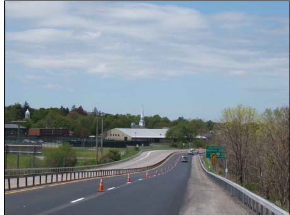
Route 8 northbound into the Village of New Hartford; the highest volume roads in Town are state roads
