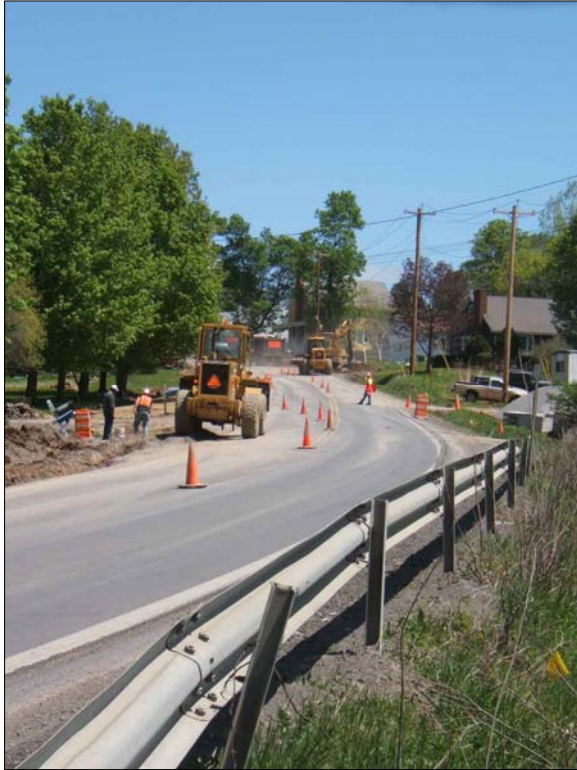
Widening of Chapman Road
